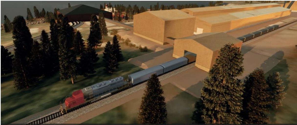
Figure 5-2 – Conceptual 3D Rendering of Rail Lines Entering Warehouse and Spodumene Concentrate Off-Load Facility
